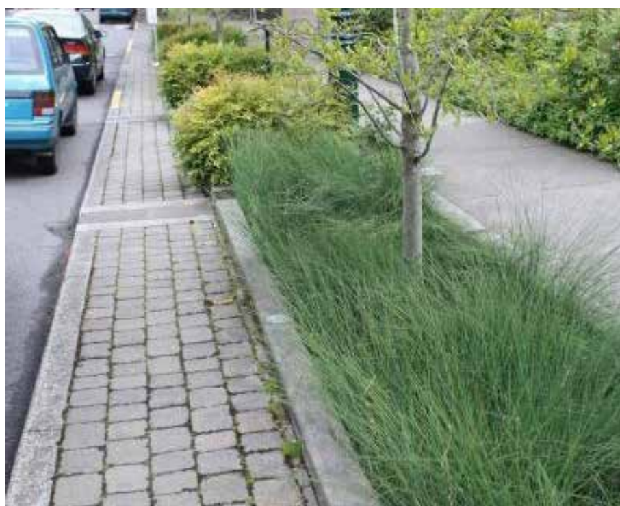
Fig. 6.29. Green street with swale
