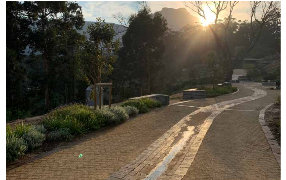
Fig. 6.65. Pedestrianised road with central drainage and indigenous fringe planting
