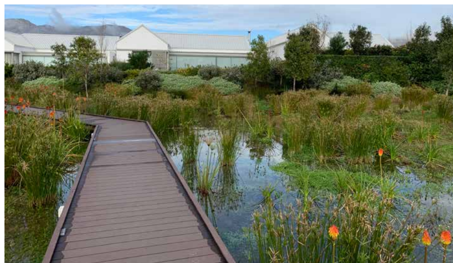
Fig. 6.74. Polishing of stormwater using endemic or indigenous planting
