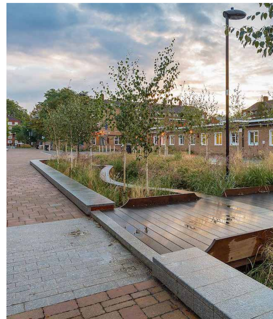
Fig. 6.31. Pedestrian oriented street and shared surface space with Sustainable Urban Drainage System / swale
